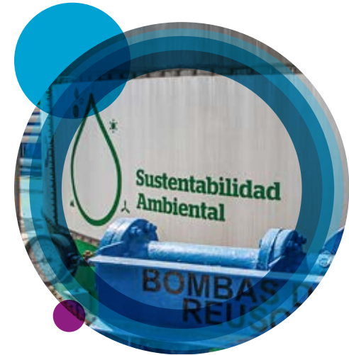
Water reuse pumps at a PepsiCo Mexico Foods facility.
